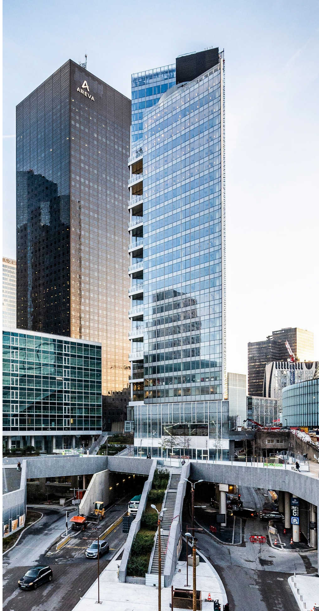
Figure 2. Trinity was designed as a comprehensive and contextual urban project for La Défense. © XXX
