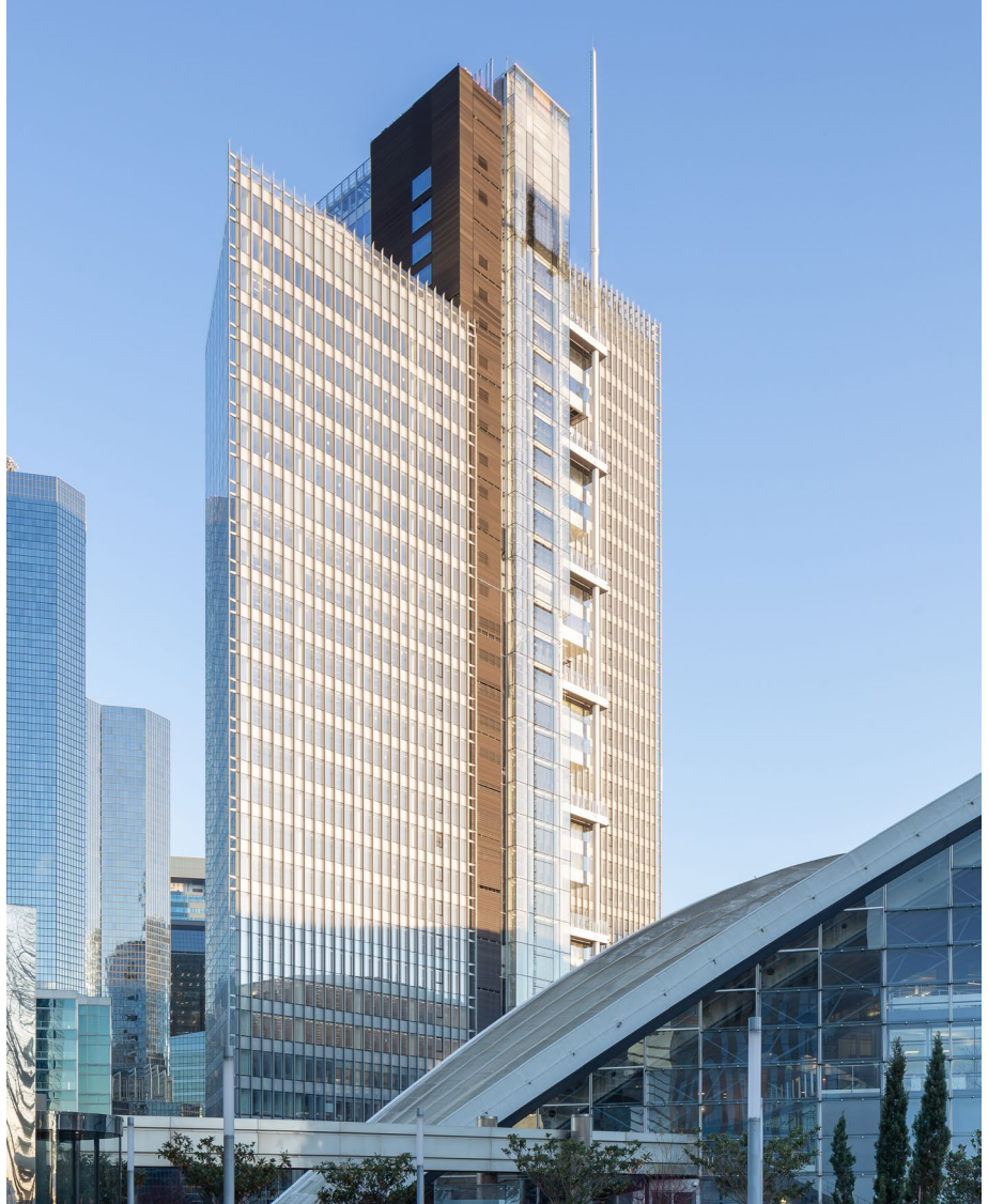
Figure 12. The façade is rendered with printed glass blades that obscure separations and aid solar protection. © Hugo Hebrard
