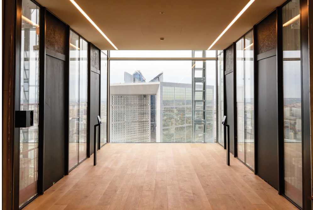
Figure 8. Elevator lobbies are bathed in light due to the transparent shaft walls and offset-core design. © Gaston Bergeret
