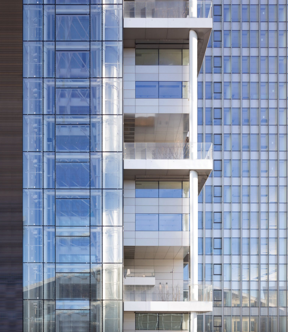
Figure 6. The offset core enabled unique design elements—a system of terraces and suspended meeting rooms, and a transparent elevator shaft. © Hugo Hebrard
